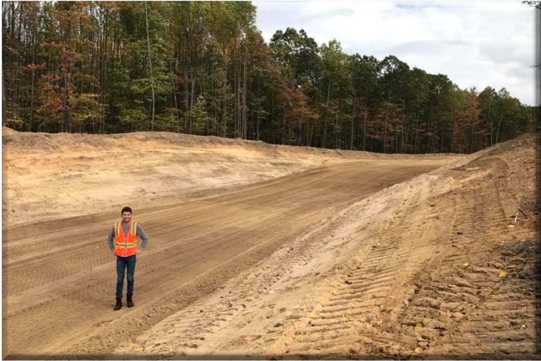
Sean Pengelly, LSRC Engineer Projects and Development, inspects the progress on extensive grading for the ARAUCO project. When completed later this year, the rail spur will include approximately 10,000 track-feet of new construction to service the new facility.
