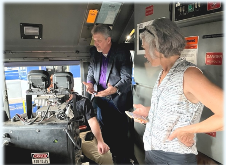
Roger Fuehring, LSRC Chief Mechanical Engineer explaining the basic functionality of an engine's controls and its operation.
