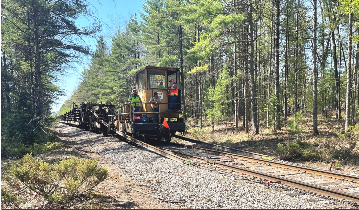
Active Unloading of New 115 lbs. Rail
